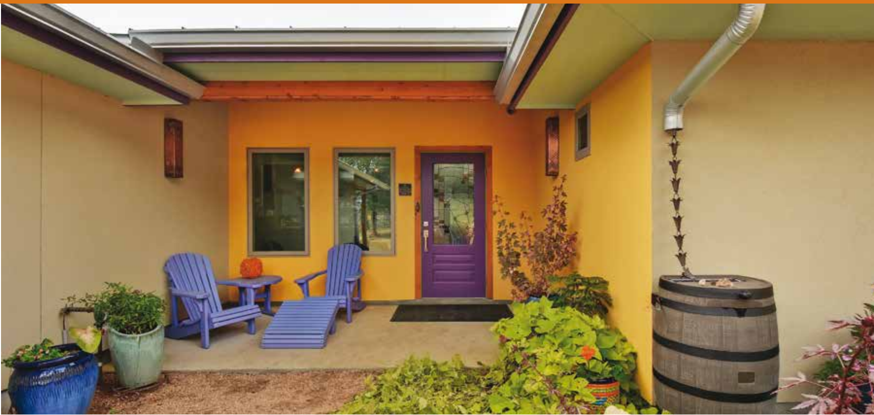
Firewise Façades. Featuring a durable stucco exterior and a Galvalume reflective metal roof, this Texas home is built and designed to local standards for wildfire resistance.
